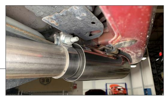
Fit the exhaust tip to the tail pipe, and slide the tip down enough to clear the rear bumper. Once clear of the rear bumper, angle the assembly upwards to allow the hanger welded to the exhaust tip to fit the vehicle rubber hanger behind the rear bumper. Secure, but do not fully tighten the exhaust clamp.
