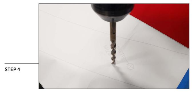
Using a 1/4" drill bit and drill, carefully drill the center of the 7mm holes and 11.5mm holes. Then finish the 11.5mm holes using a 1/2" drill bit. Use touch up paint to cover any exposed metal. Ensure the surface is clean and free of any metal debris prior to installing the spoiler.
